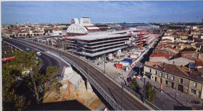
Extension of the Bordeaux Saint-Jean station: the Belcier building
