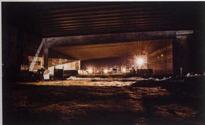
Boring the Guit Bridge. A large-scale lighting operation
