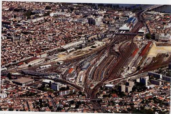
The Aquitaine Technicentre water systems
