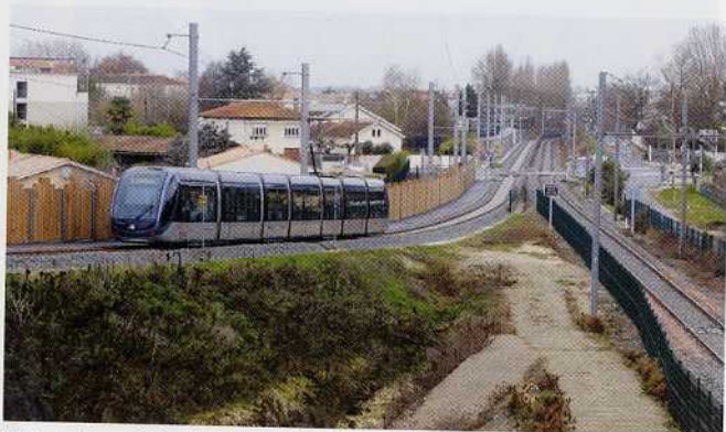
Extension of Bordeaux tram line C
