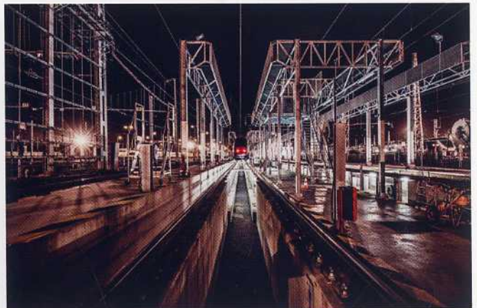
The Bordeaux TGV maintenance station
