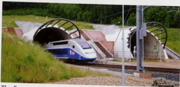
The Saverne tunnel
